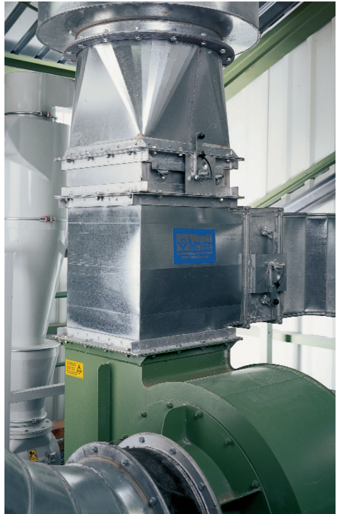
High-efficiency centrifugal fan with changeover for return or exhaust air
