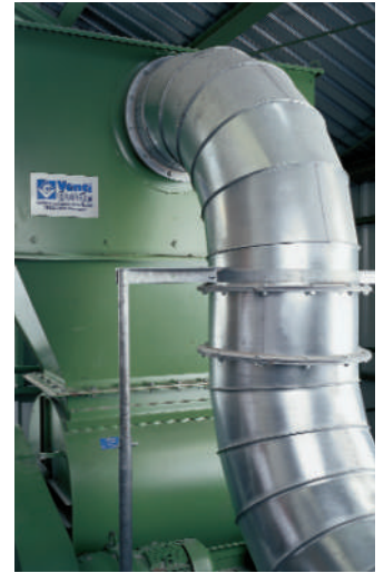
Separator with discharge through airlock
